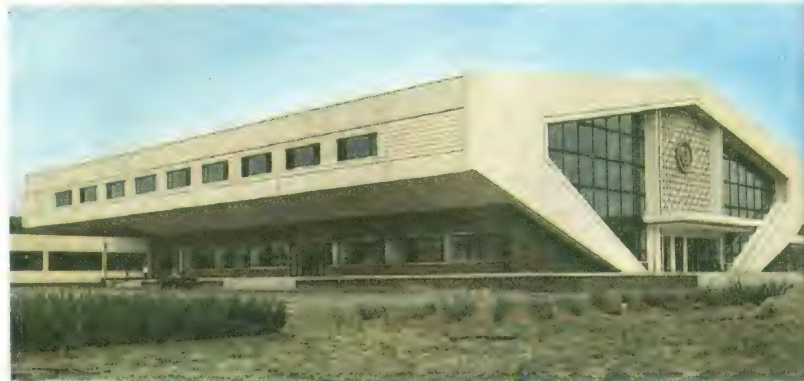
청춘거리 종합기관 The Combative Sports Gymnasium in Chongchun Street →
